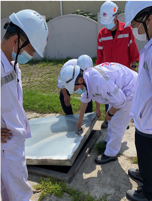
Hidden risk inspection
