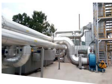
惠陽塗料廠房的VOC處理設施 Huiyang coatings plant's VOC treatment facility
