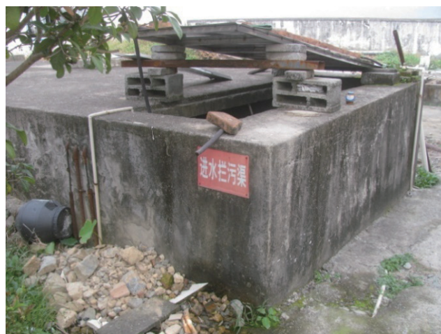
Wastewater filter and disposal system
