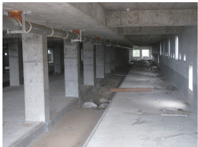
Construction of nullah within pig barns
