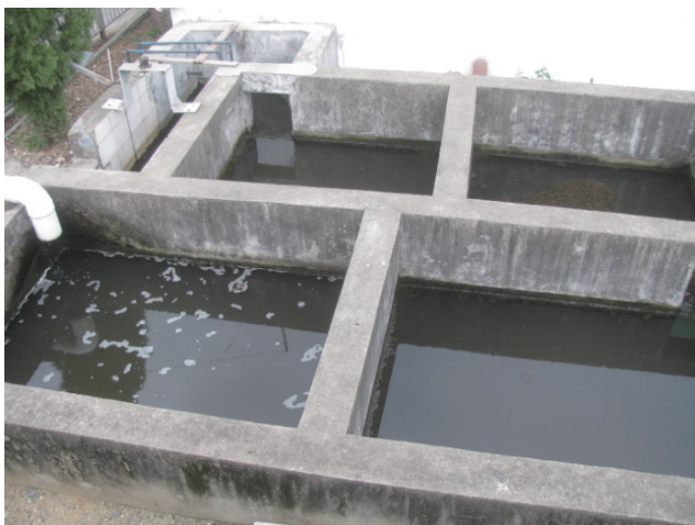
Wastewater filter and disposal system
