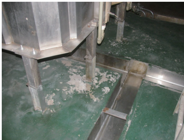
Gutters within slaughterhouse for waste water drainage
