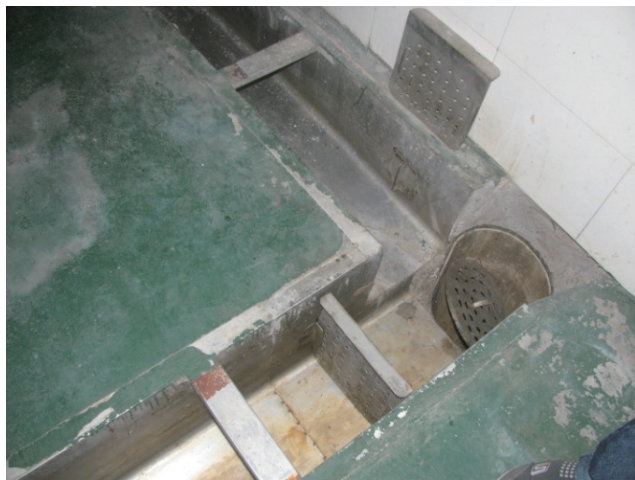
Gutters within slaughterhouse for waste water drainage
