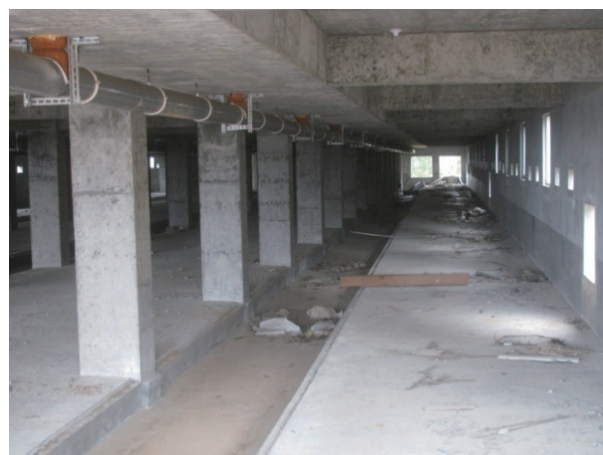
Construction of nullah within pig barns
