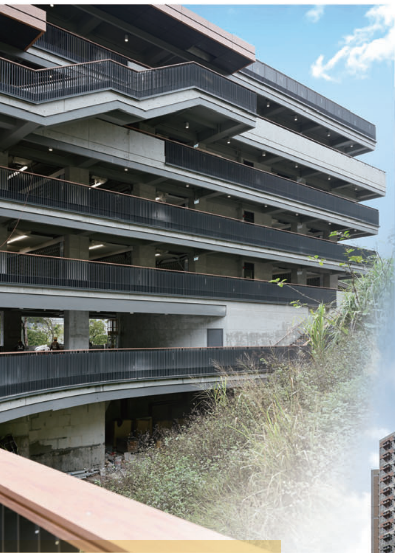
Construction of Columbarium at Wo Hop Shek Cemetery — Phase 1 和合石墳場靈灰安置所第一期 興建工程
