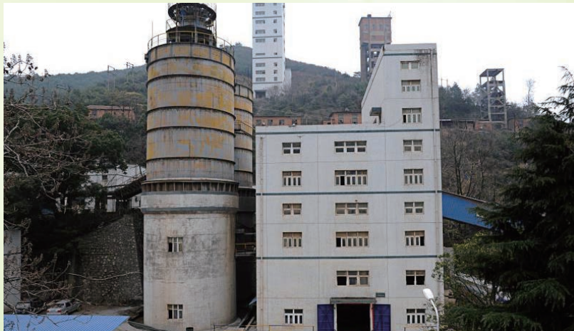
Cemented Filling Station at Wushan Copper Mine
