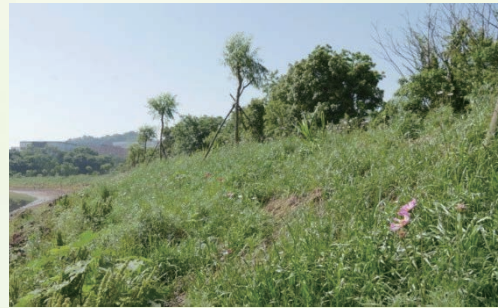
Ecological Restoration Project on Open Areas Surrounding the Lake on the West of the Mining Area
