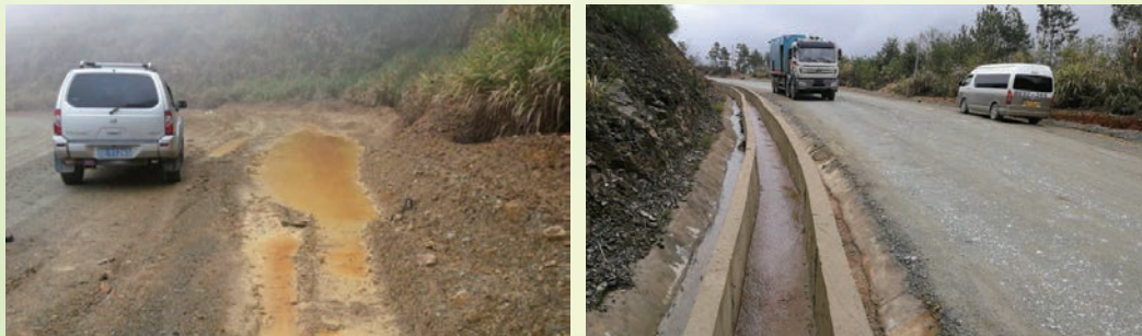
Comparison before and after the Clean Water and Sewage Diversion Project on Fujiawu Access Road
