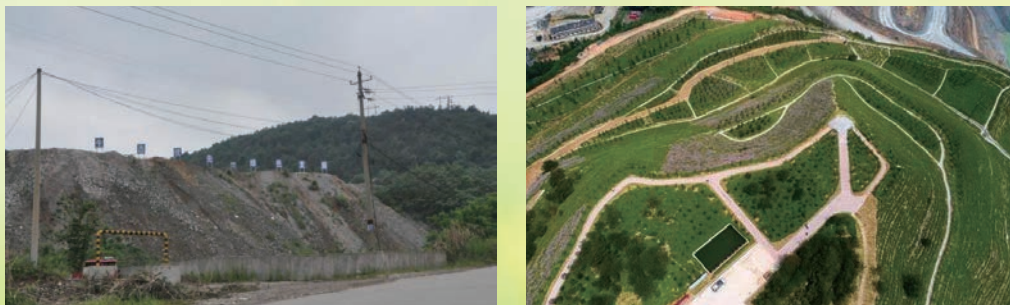
Comparison before and after Land Reclamation
