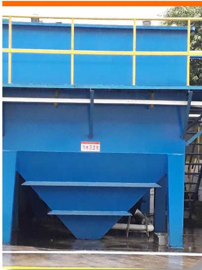
The pictures above show the sewage sedimentation tank (left) and the sewage facility (right).
