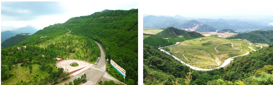
The botanical garden and flower and fruit garden of the Zijinshan Gold and Copper Mine after conducting improvement work at the dumping yard
