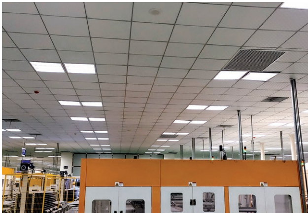
Using LED lights instead of fluorescent lamps in workshops 車間使用LED燈取代螢光燈
