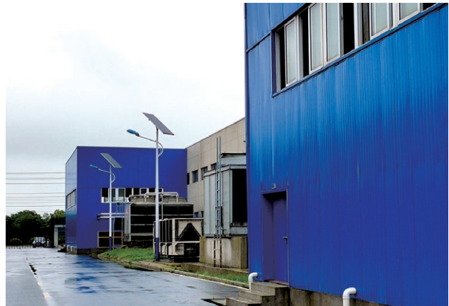
Outdoor solar street lights 室外太陽能路燈
