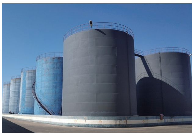
The oil tanks before renovation 油罐改造前
