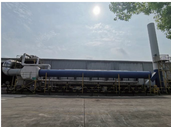
VOCs and ammonia collection and treatment systems VOCs及氨氣收集處理系統
