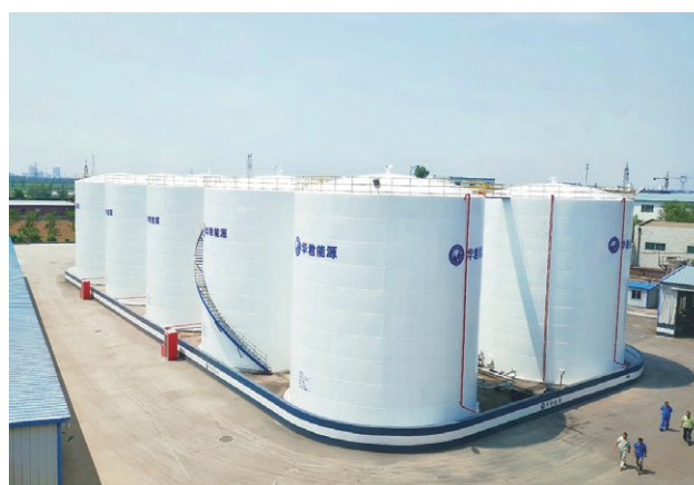
The oil tanks after renovation 油罐改造後
