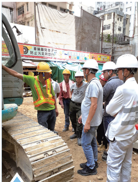
4 Site safety inspection
