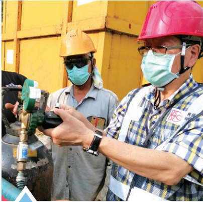
1 Training conducted on site
