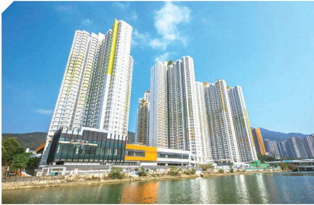
Public Rental Housing Development Phase 2 in Shek Mun
