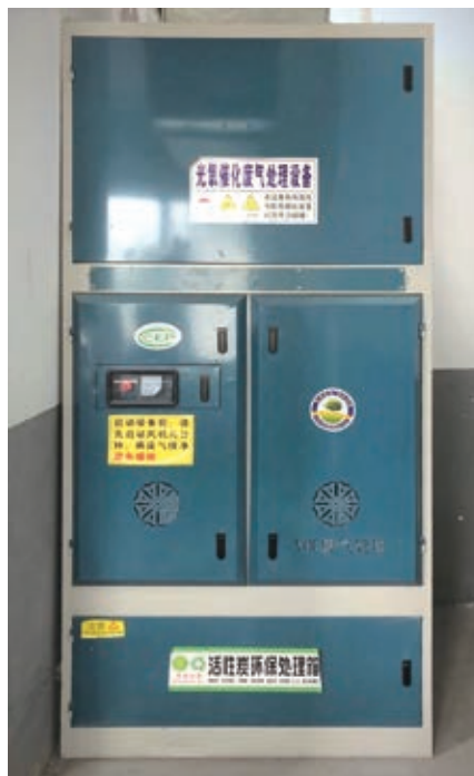
Figure 5: Photocatalytic oxidation treatment facility in Changzhou Repair Shop
