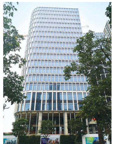
Construction of BEA's GBA Headquarters in Qianhai, Shenzhen is expected to complete in 2021. 東亞銀行位於深圳前海的大灣區總部預計將於2021年落成。
