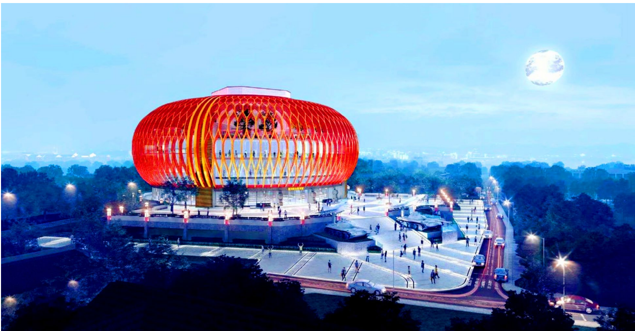
四川成都建川綜合陳列館鋁合金網殼結構建設項目 Aluminium alloy reticulated shell of Comprehensive Exhibition Hall in Chengdu, Sichuan
