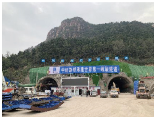
Note: The construction site of Xinxiang-Jincheng Expressway
