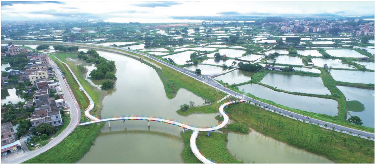
鹤山市沙坪河综合整治工程PPP项目整治后 PPP project of the comprehensive improvement work of the Shaping River (after improvement) in Heshan city
