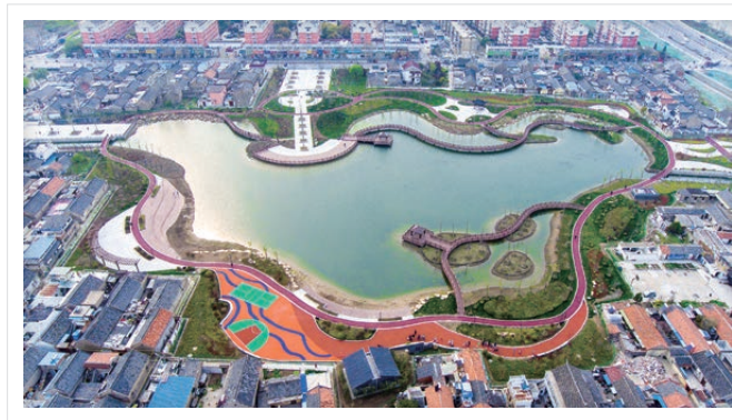
整治后的淮安黑臭水体综合整治项目 Comprehensive improvement project of Huai'an black and odorous water after improvement
