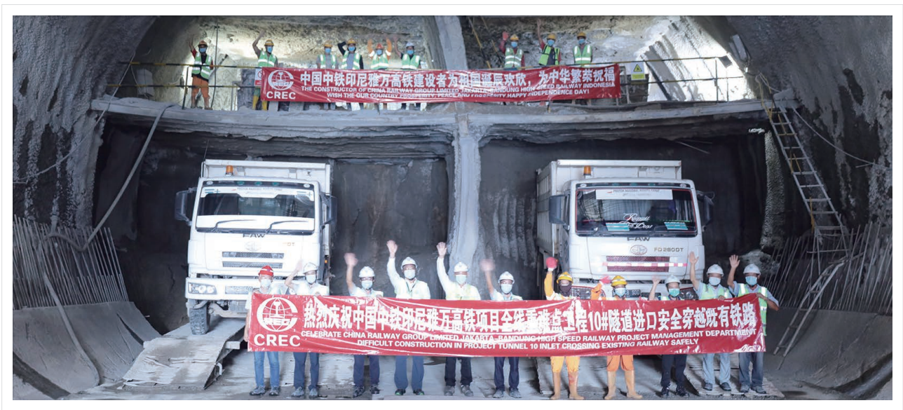
中国中铁印尼雅万高铁项目10号隧道顺利穿越既有铁路礼 Ceremony of the breakthrough in No. 10 tunnel of the Jakarta-Bandung high-speed railway project undertaken by CREC
