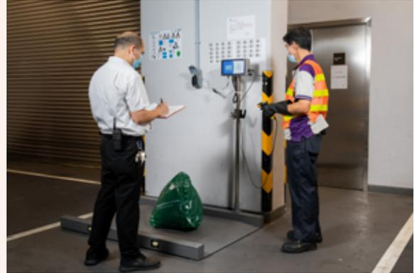
At both properties, smart scales are embedded in the systems to capture the disposal time, type of waste and weight. Data is then collated and made available through a mobile application.
