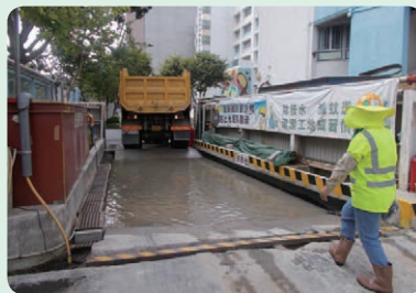
Vehicle Wheel Washing 車輪清洗
