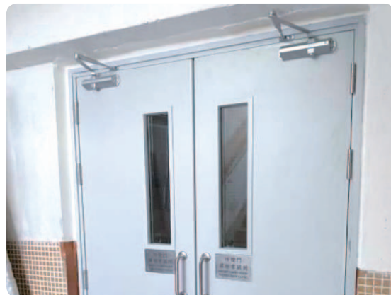
After Repair 維修後
