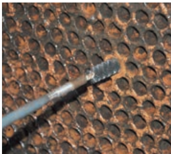
Figure 2-1: Traditional cleaning of the condenser of the ice water machine before improvement
