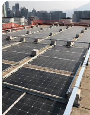
Solar Panels Installed at Roof of MTR Headquarters Building
