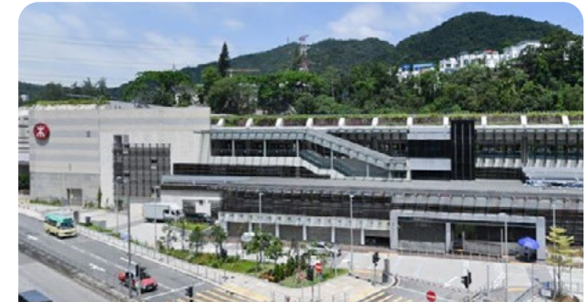
Design of Hin Keng Station features wood and brown colours to blend with the surrounding environment
