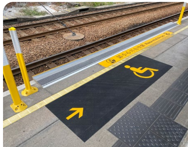
We use Board Easy Mat to enable wheelchair users to easily board and alight our LRVs
