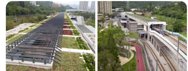
Around 5,000 square metres green roof atop Hin Keng Station and its associated structures
