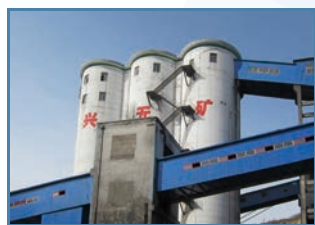
Xingwu Coal Mine 興無煤礦
