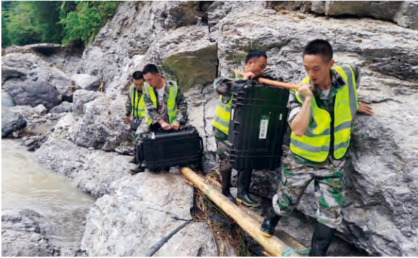
■ Our workers at Meishan subsidiary hiked 10 kilometers carrying 100 kg of equipment to repair the communications network
