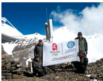
■ In November 2007, China Mobile opened a base station on Mount Qomolangma at an elevation above 6,500 meters
