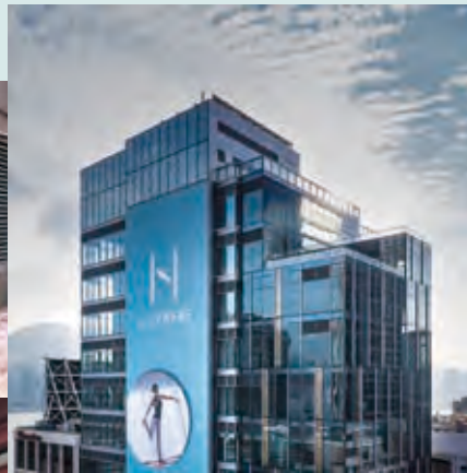
H Zentre, Tsim Sha Tsui, Hong Kong
