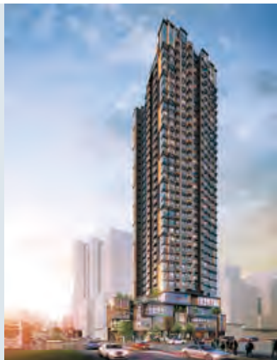
Castle Peak Road/Un Chau Street Project, Sham Shui Po, Hong Kong (artist's impression)
