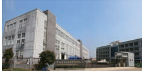
Plant after Renovation
