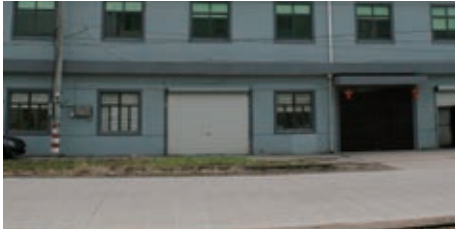
Plant before Renovation
