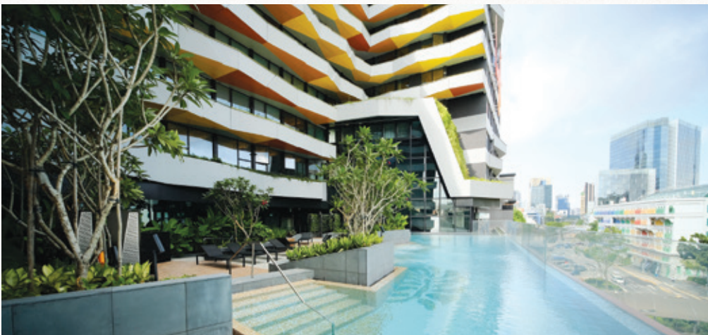
TFX Funan (新加坡) — 游泳池及休閒甲板 TFX Funan (Singapore) — Swimming Pool With Relaxation Deck
