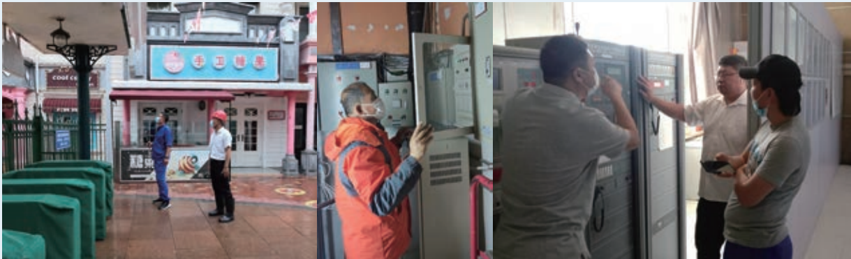
Safety inspections in the park 園區安全檢查工作
