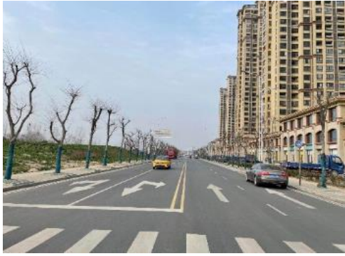
Lu'an Branch - Municipal Road PPP Project in Huoqiu County
