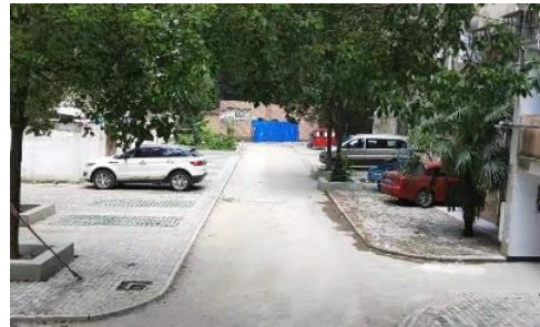
Tongling Branch - Old Communities in Tongling after renovation
