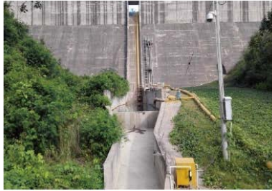
Wastewater outlet and online monitoring system of the Zijinshan Gold and Copper Mine
