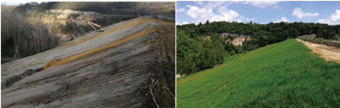
Comparison of the slope of Zijin's tailings storage in Serbia before and after ecological restoration
