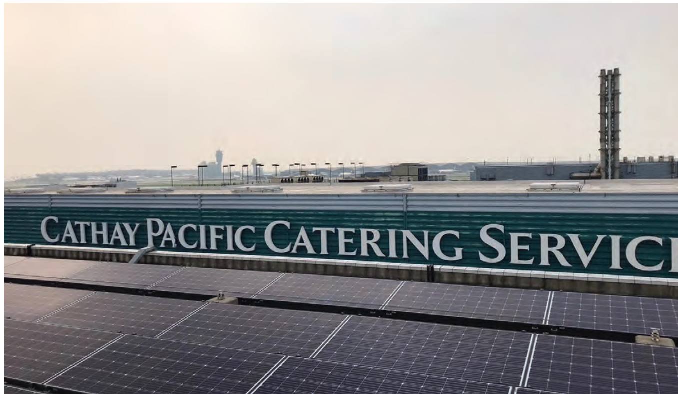
Solar panels on the rooftop of Cathay Pacific Catering Services' headquarter building
