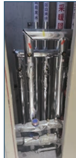
Winterizing fire sprinkler system
