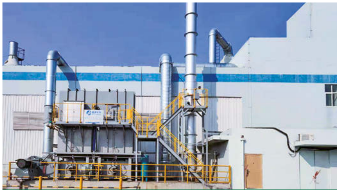
Volatile organic compound treatment facilities were employed at the Qingdao Likang Factory
