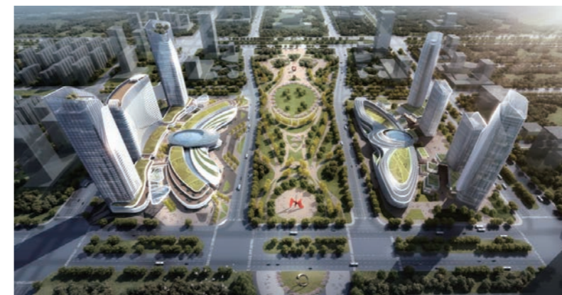
◆ JK Institute undertook the geotechnical engineering survey projects of Greenland Silk Road Global Trade Port and supporting projects. Greenland Silk Road Global Trade Port will be a national import and export platform and financial center of the 'Belt and Road', providing one-stop services of commodity trade and supply chain support for global enterprises.
