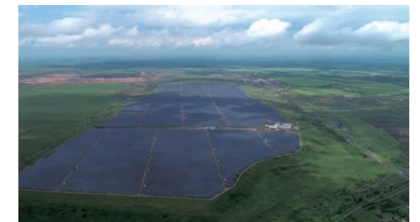
◆ 200 MW PV Power Plant Project in Nikopol, Ukraine
