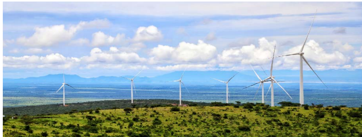
◆ 102 MW wind power project in Kipeto, Kenya
