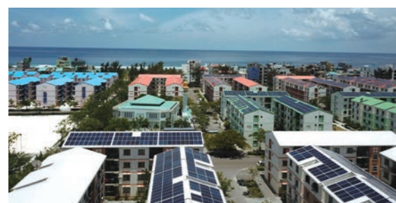
◆ Maldives 1.5MW PV power plant project
