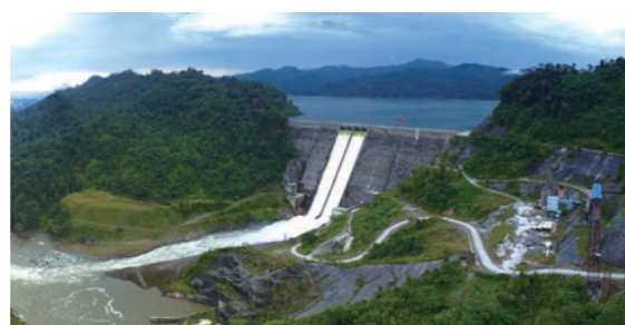
◆ Murum Hydropower Station Project in Malaysia
