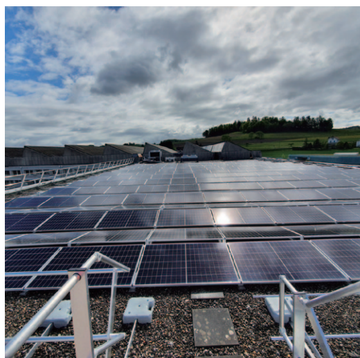
In Murten, Switzerland the Group installed 900m 2 of photovoltaic cells on the roof of the factory, generating an estimated 123 MWh per year.
