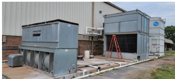
Maintenance work and improvements to chillers and other HVAC systems resulted in a 43% reduction in water consumption from FY19/20 to FY20/21 in Springfield, USA
