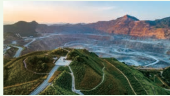
楊桃塢230標高排土場部分邊坡生態恢復工程實施效果 Implementation effect of ecological restoration project of partial slope of dump at elevation 230 of Yangtaowu
