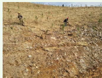
覆蓋草簾 Covering grass curtains
