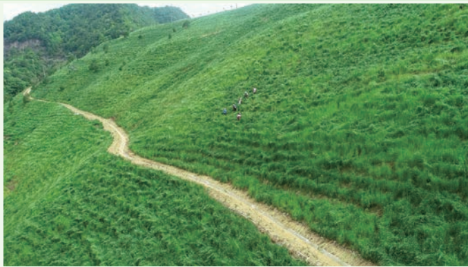
富家場500標高排土場部分邊坡生態恢復工程實施效果 Implementation effect of ecological restoration project of partial slope of waste dump at elevation 500 of Fujiawu
