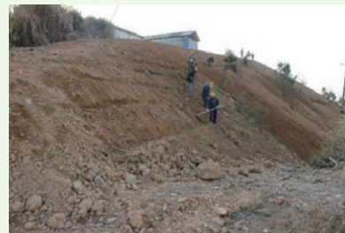
開挖種植條溝 Excavation of planting strip trench
