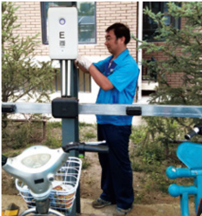
Installing EV Charging Piles
