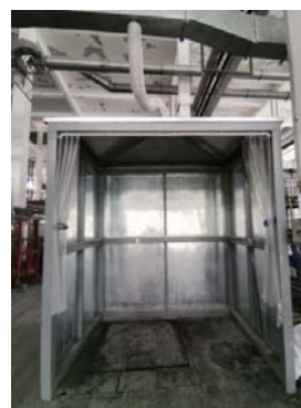
(Installing exhaust gas collection facilities in hazardous waste depots and weighbridge batching areas)
