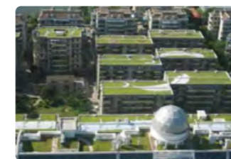
屋頂綠化減少下墊面熱量聚集 Green roof reduces underlying heat accumulation
