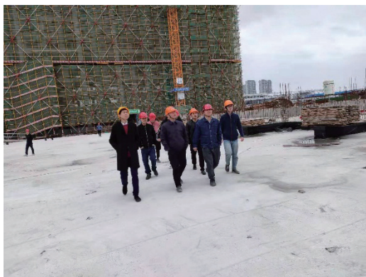
Weekly safety on-site inspection 每周安全現場巡查
