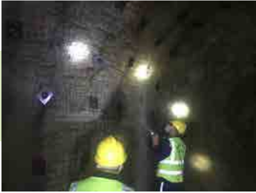
Jiama organized underground on-site safety inspection.
