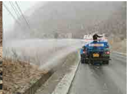
Jiama Mine rented two waterwheels to carry out greening and watering in the spray planting area every day.
