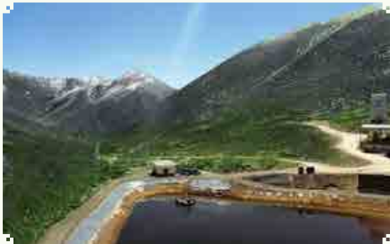
Jiama Mine launched Sibugou backwater project.
