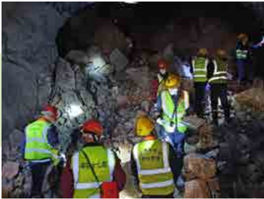
Jiama conducted monthly safety inspection.
