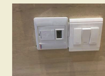
Upgrade of LED time-controlled system, acousto-optic system and radar sensing system
