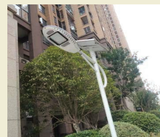
Solar high-pole lamps
