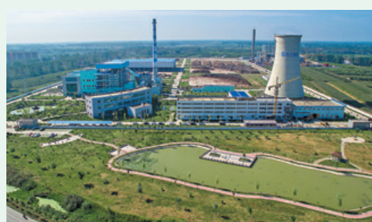
Dangshan Integrated Biomass and Waste-to-energy Project 蕩山生物質及垃圾發電一體化項目
