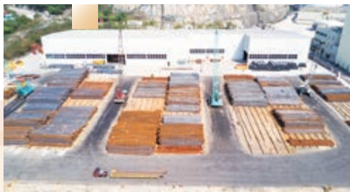
Automated Rebar Processing and Assembly Plant 自動化鋼筋加工及裝配廠
