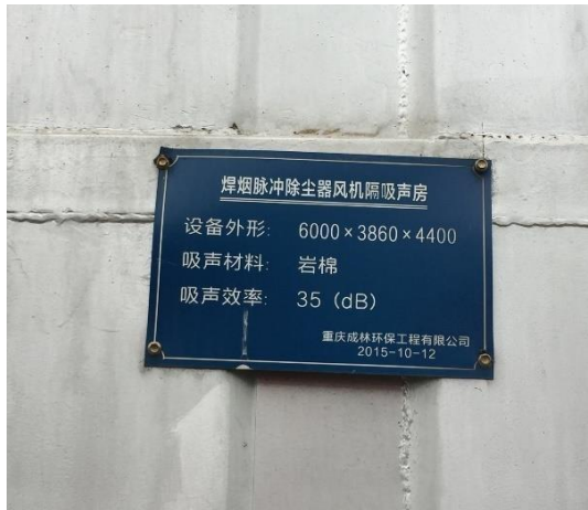
Figure 2 Physical Sound Insulation Measure—Noise Absorption Room
