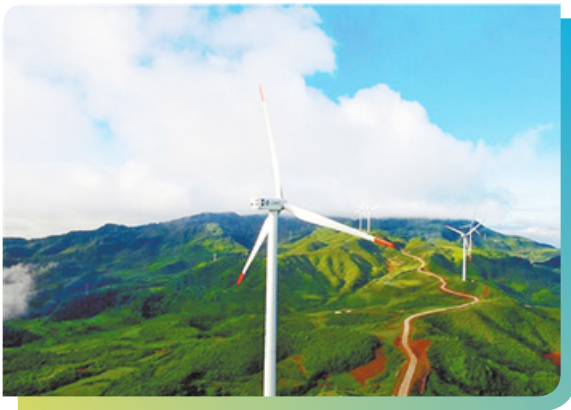
Modou Mountain Wind Farm, an entrusted management project of CGN New Energy
