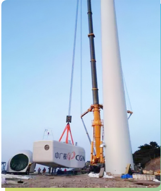
Wind turbine hoisting at the Taigu Fancun Wind Power Project
