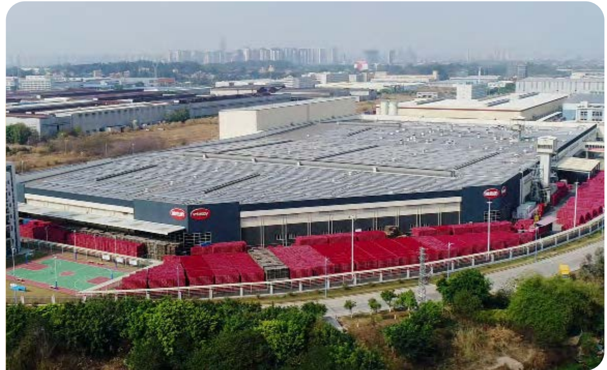
Rooftop solar panels at our Foshan manufacturing plant
