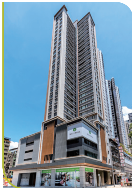
West Park at Nos. 256-258 Tung Chau Street 位於通州街256號至258號之West Park
