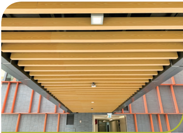
Supply and installation of suspended ceiling system at balcony and podium level for redevelopment at No. 3 Marble Road, North Point 北角馬寶道3號之重建項目—供應及安裝露台及平台層之假天花系統
