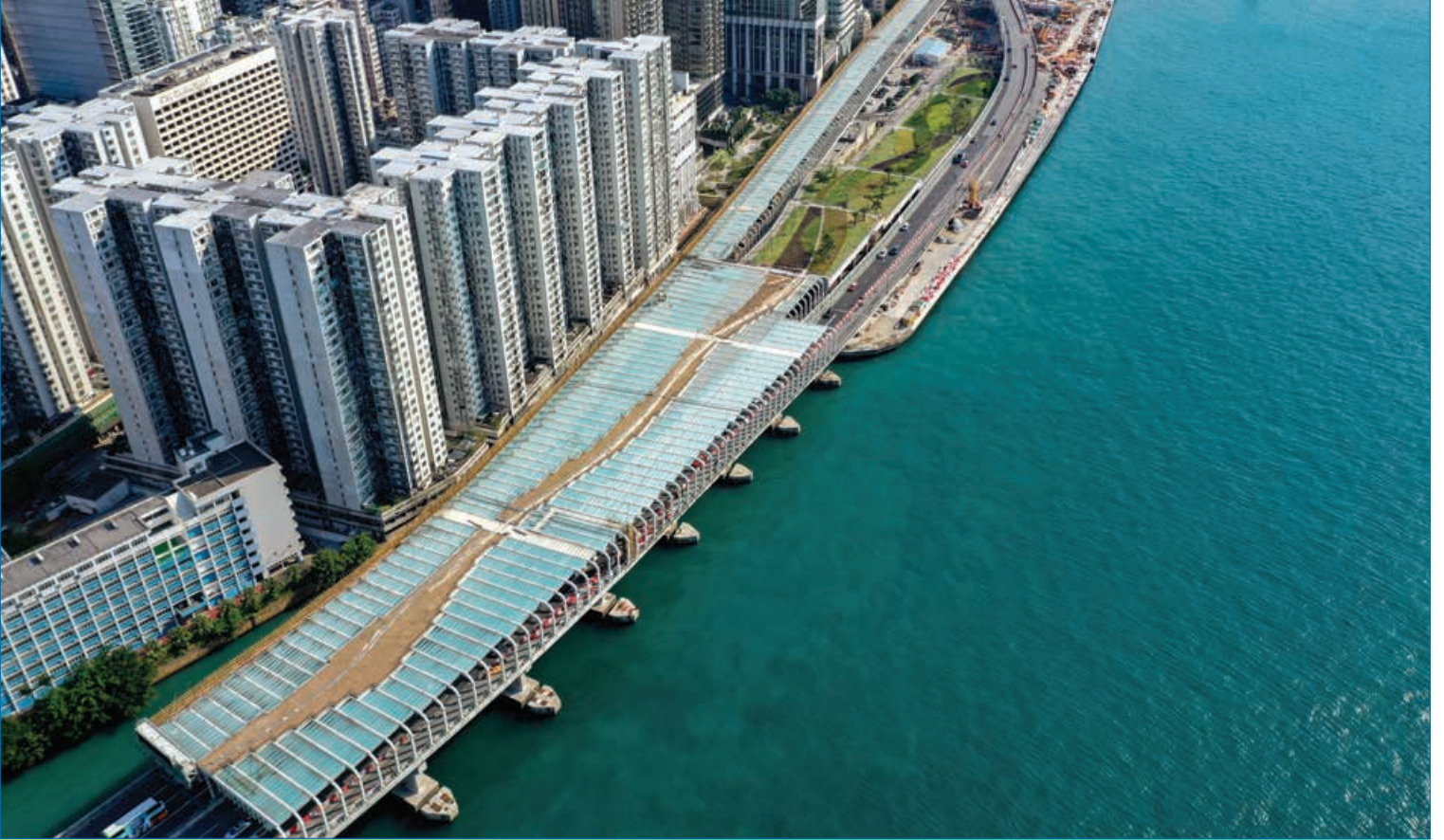
Central-Wan Chai Bypass: Tunnel (North Point Section) and Island Eastern Corridor Link 中環灣仔繞道：北角段隧道和東區走廊連接路工程
