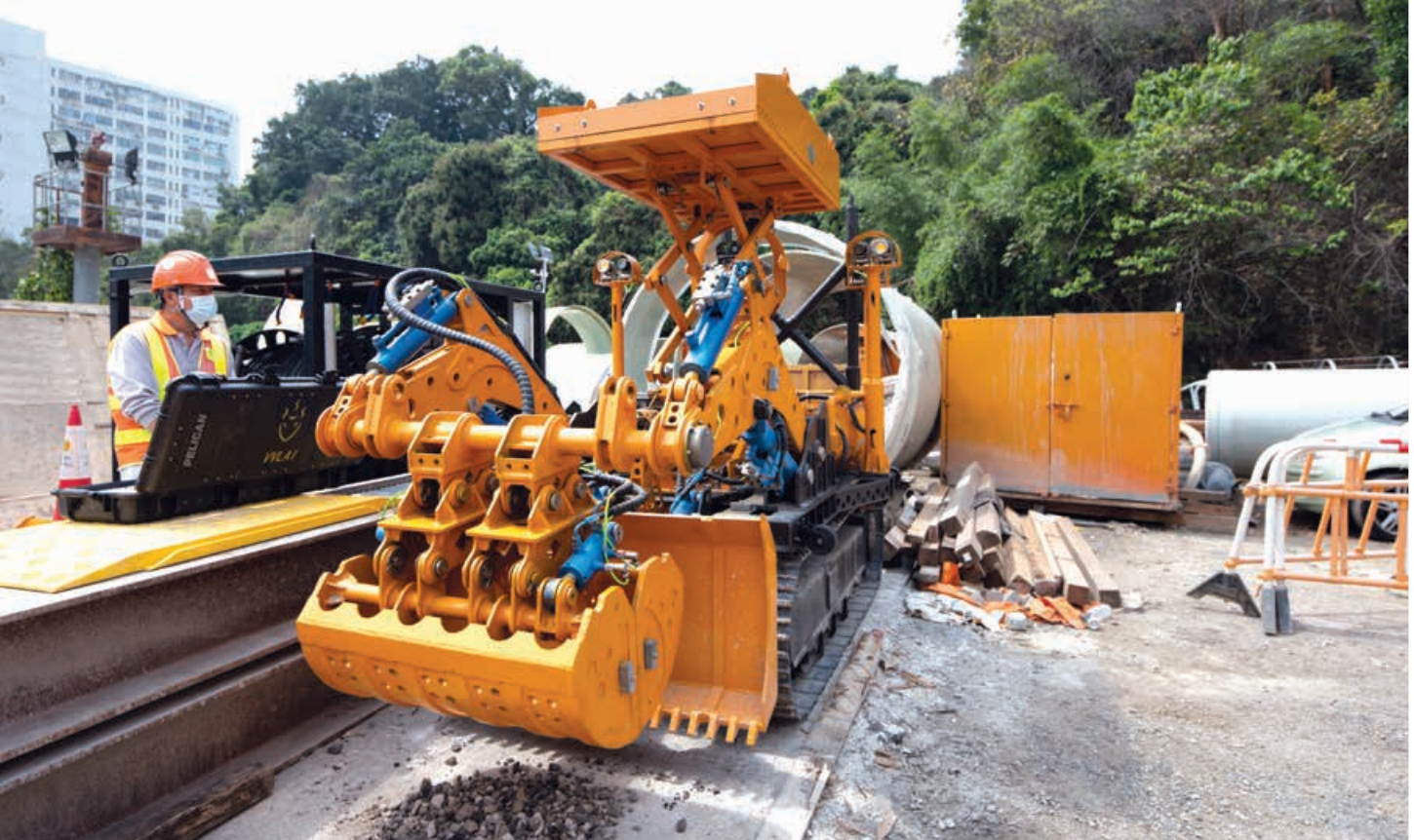
Rehabilitation of Trunk Sewers in Tuen Mun 屯門污水幹渠修復工程
