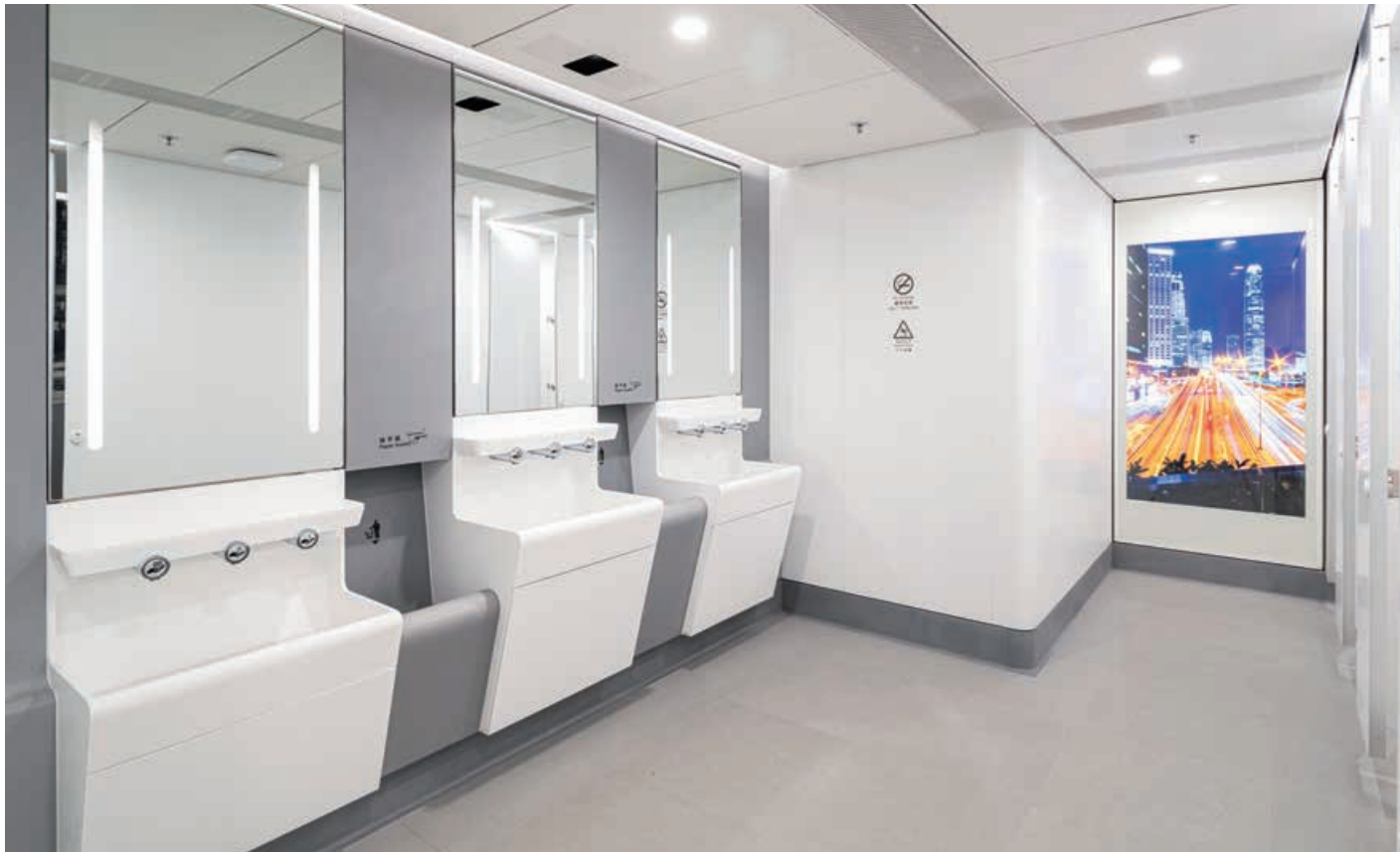
Revamp of Public Toilets at Terminal Buildings at Hong Kong International Airport 香港國際機場客運大樓公共洗手間翻新工程
