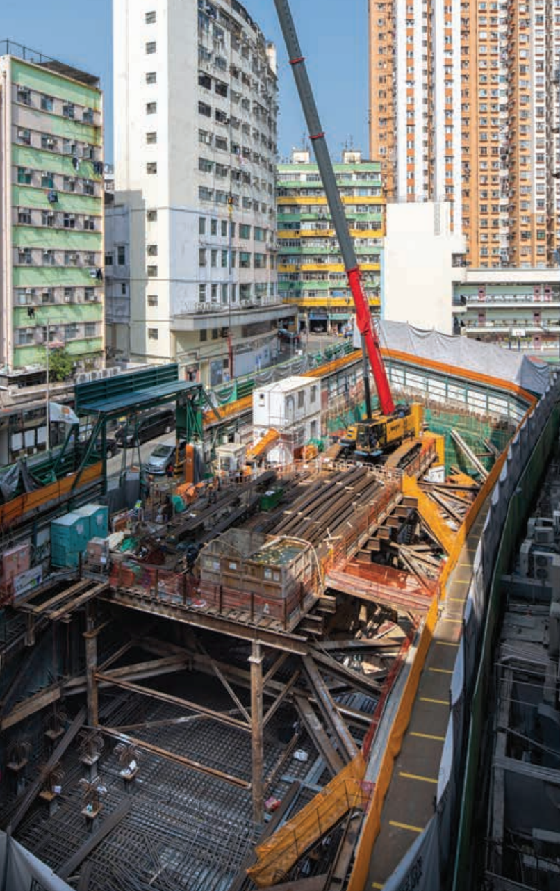
Main Contract for the Proposed Composite Development at Nos. 12–30 Hang On Street, Kwun Tong, Kowloon 九龍觀塘恒安街12至30號綜合用途房屋建造工程
