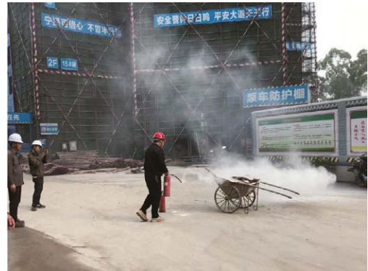
Demonstration of the Proper Use of Fire Extinguishers 示範正確使用滅火筒
