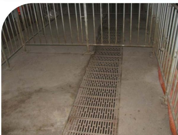
Covered nullah within pig barns for pig waste collection and drainage
