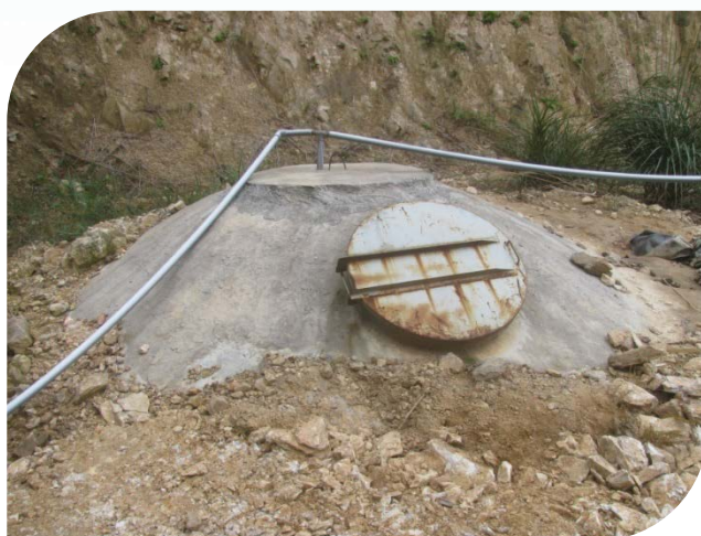
Self digestion enclosed pit for dead hog disposal
