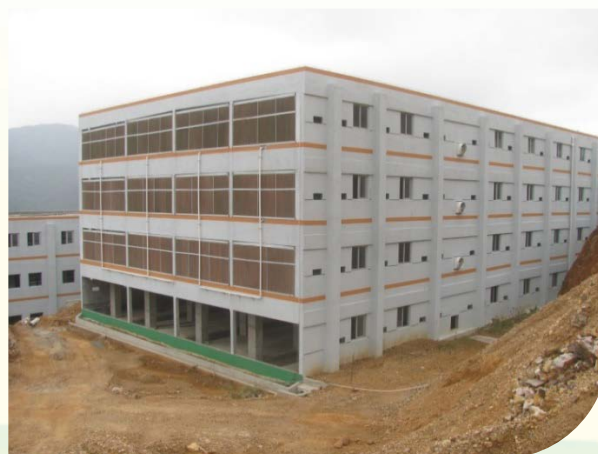
Construction of pig barn with adequate ventilation
