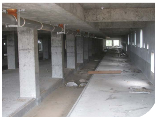
Construction of nullah within pig barns
