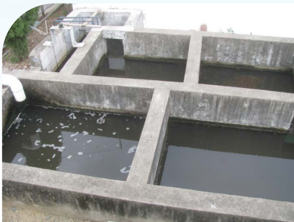
Wastewater filter and disposal system
