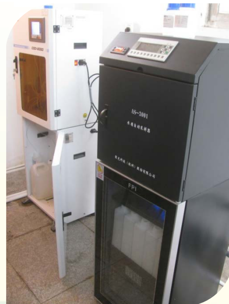
Treated waste water monitoring system
