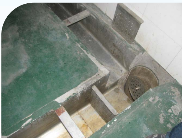
Gutters within slaughterhouse for waste water drainage
