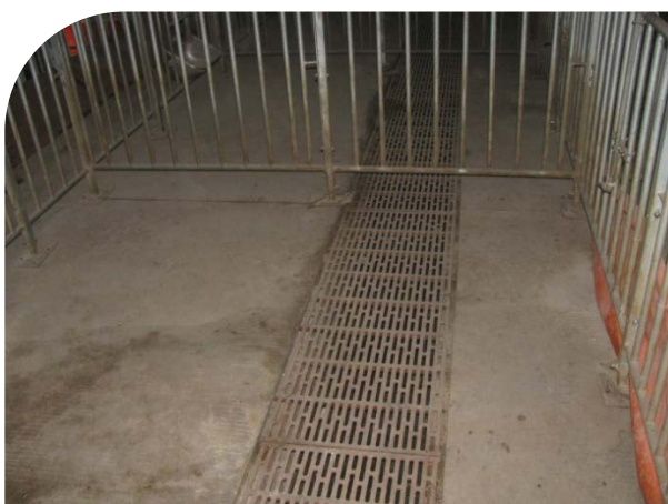
Covered nullah within pig barns for waste water drainage
