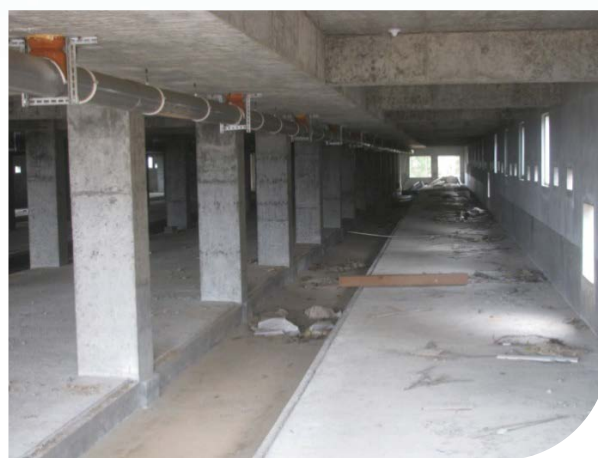
Construction of nullah within pig barns
