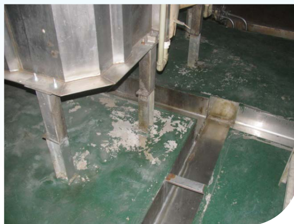
Gutters within slaughterhouse for waste water drainage
