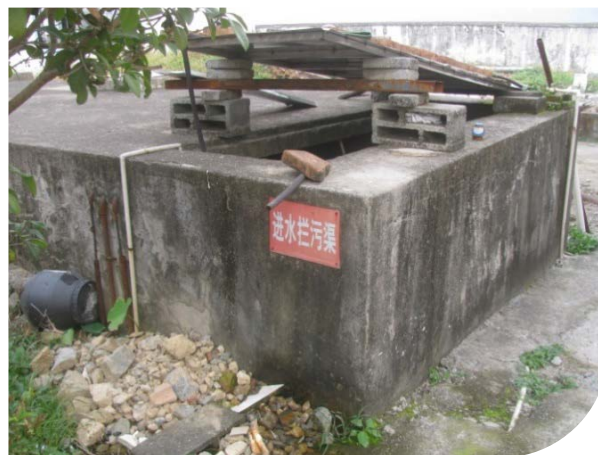
Wastewater filter and disposal system
