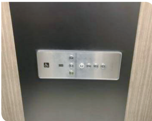
Elevator buttons at reachable height
