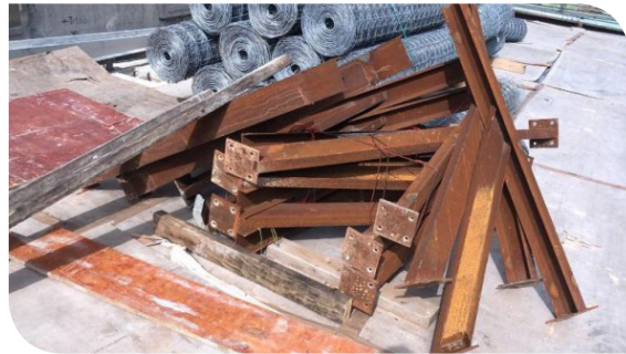
Metal collected at the construction site for recycling
