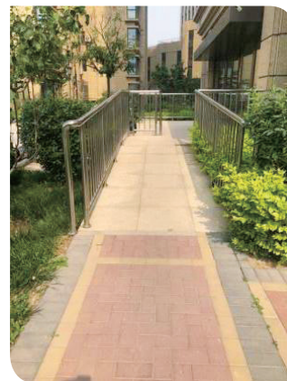
Accessible ramp and pathway
