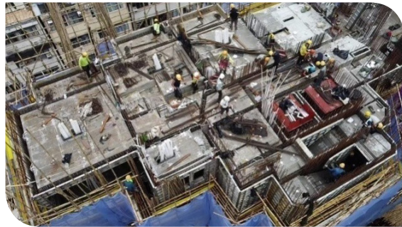
Aluminium formwork used for the construction of typical floors to reduce timber use
