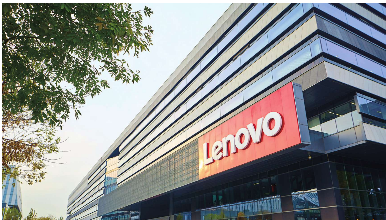
Lenovo's operation center in Beijing, China.
