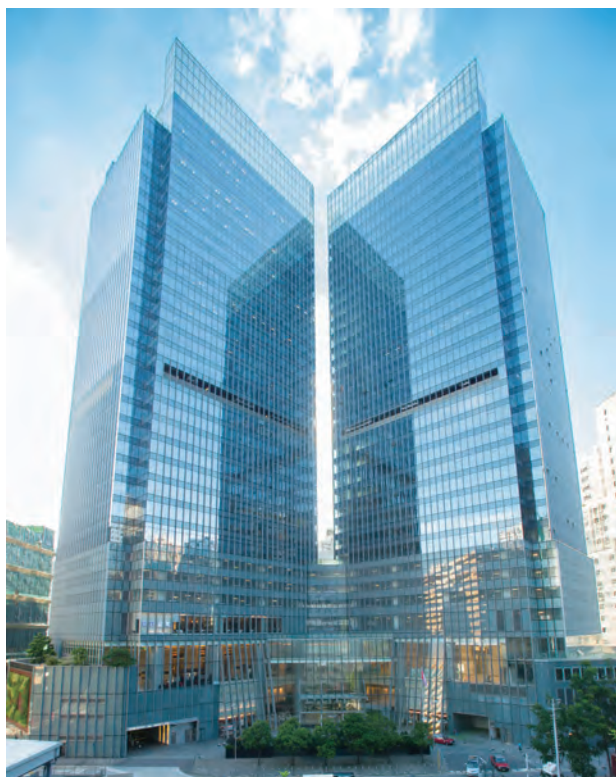
○ KCC, Kwai Chung, Hong Kong
