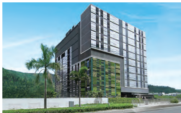
○ MEGA Plus, SUNeVision's data centre in Tseung Kwan O, Hong Kong
