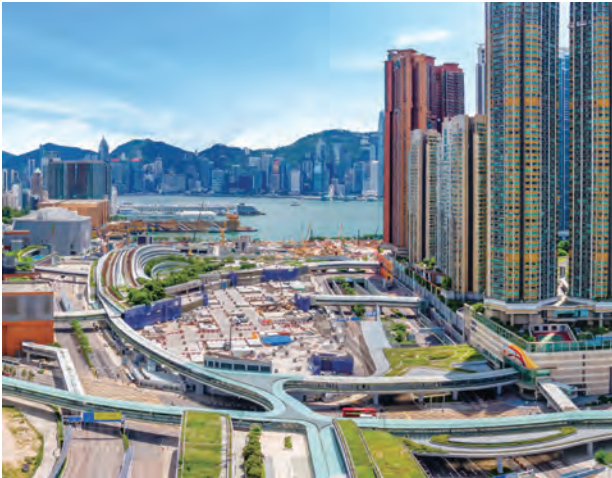
○ High Speed Rail West Kowloon Terminus Development
