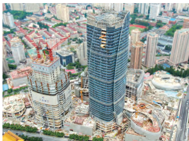
○ The two iconic office towers of ITC, Shanghai under construction
