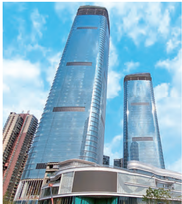
○ Chengdu ICC, Chengdu
