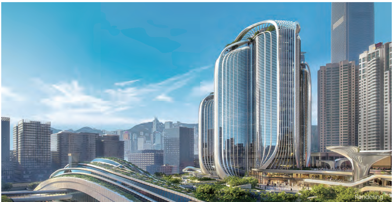
○ High Speed Rail West Kowloon Terminus Development
