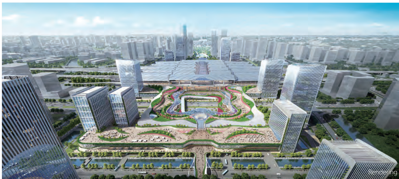
○ Guangzhou South Railway Station project, Guangzhou
